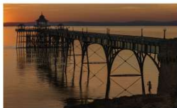
Underneath the Pier Peter Tulloch ARPS DPAGB
